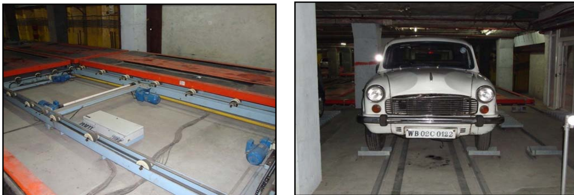
Figure 10.3: Types of Parking: a) Palette Shifting and b) Shuttle
