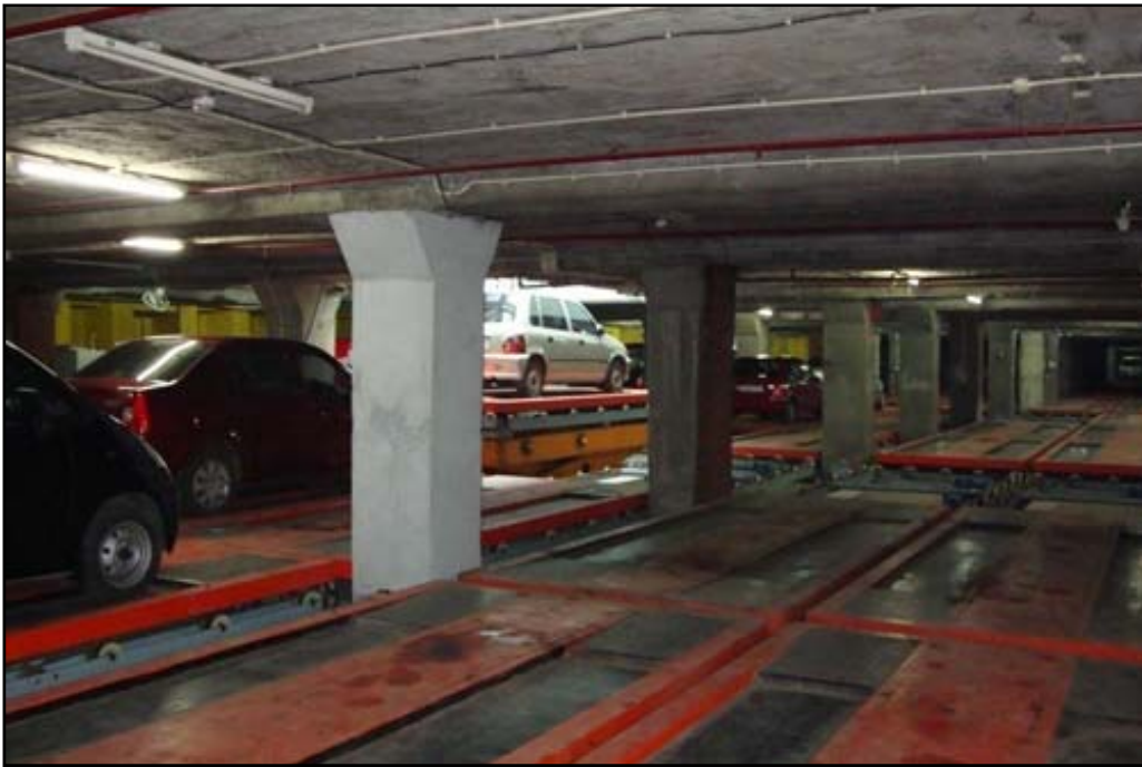
Figure 10.4: Underground Parking Bay that can accommodate 250 cars in 5 blocks
