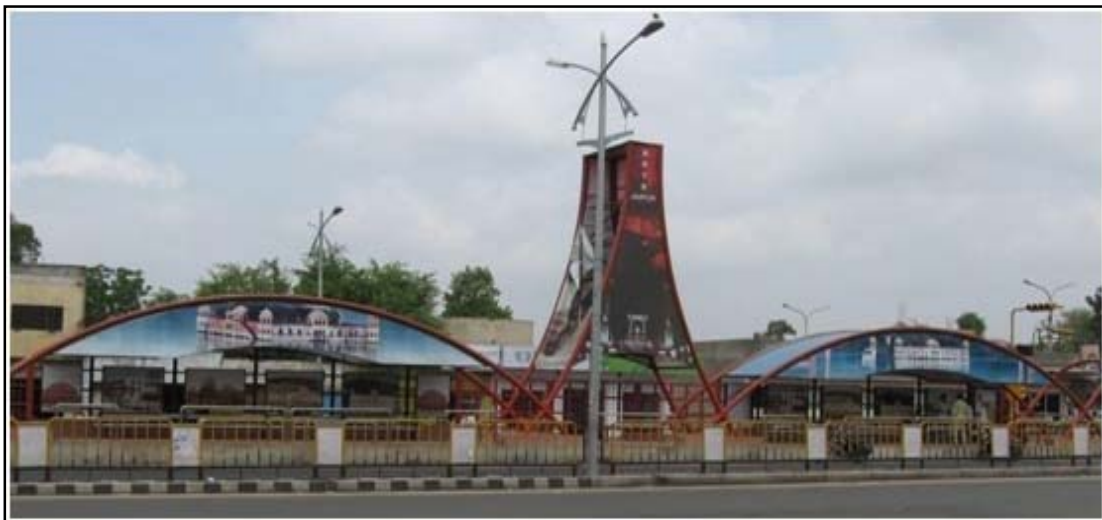
Figure 3.3: View of Bus Station / Stop on BRTS Corridor
