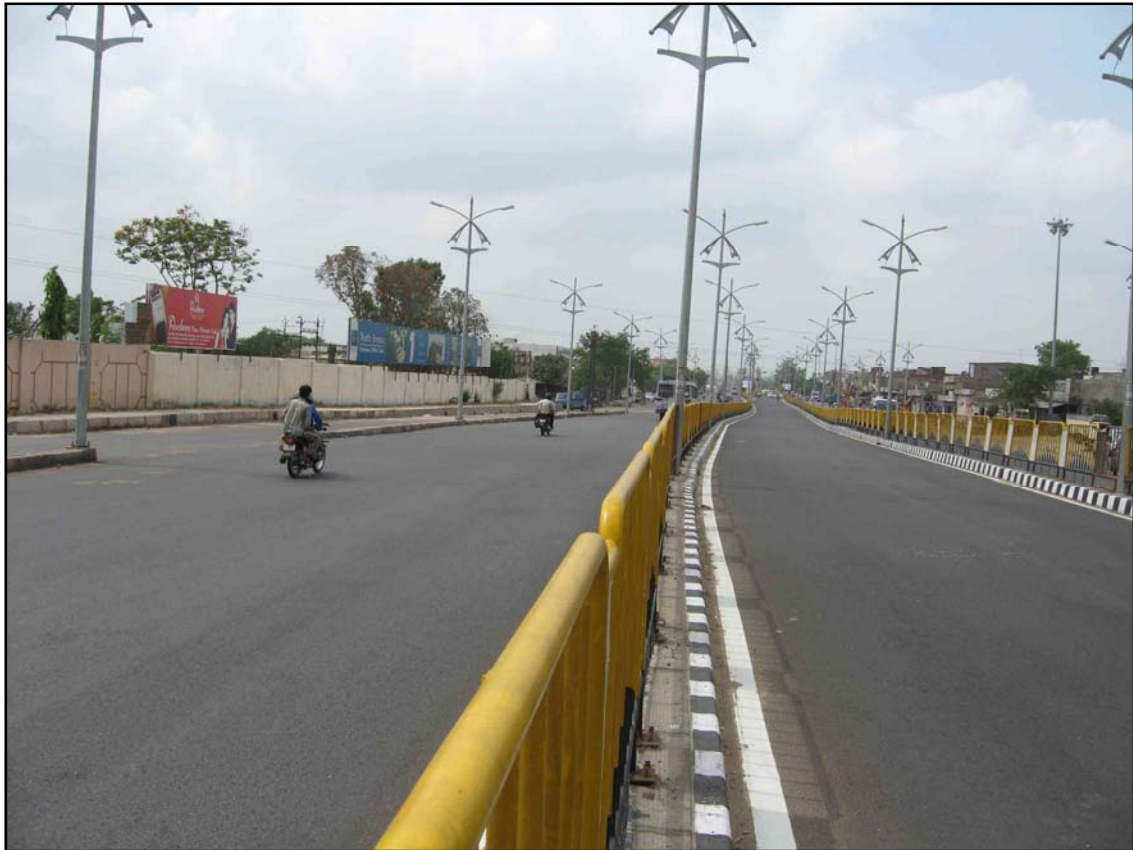
Figure 3.4: BRTS corridor having side lanes and footpath on both the side
