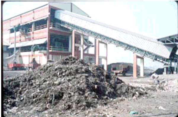
Photo 5: Solid Waste Treatment Plant Through PPP in Ahmedabad
